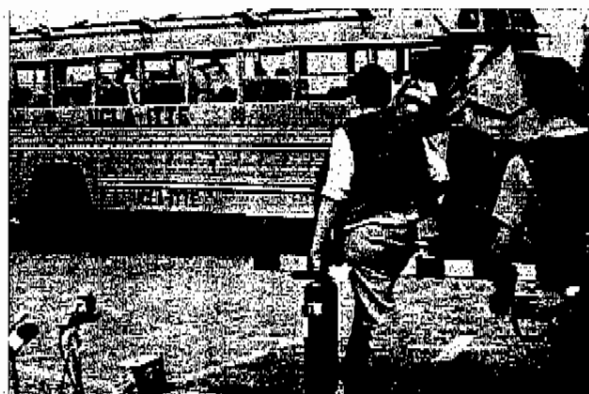
Fig. 16(b) - Thirteen-year-old lands on driver at 1250 ms. Smoke from a post-crash fire starts to enter passenger compartment on right. Prompt action by UCLA crew extinguished this engine compartment fire eliminating hazard to passenger compartment. An important consideration is the almost hopeless problem of promptly evacuating a bus load of unconscious and dazed children through inadequate escape routes
