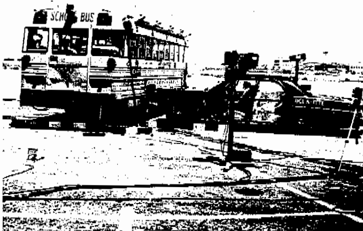
Fig. 86(a) - Traveling 60 mph, a 1966 Chevrolet contacts right-rear dual wheels of 1965 GMC-Superior bus
